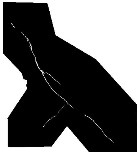
Automatic fault detection
